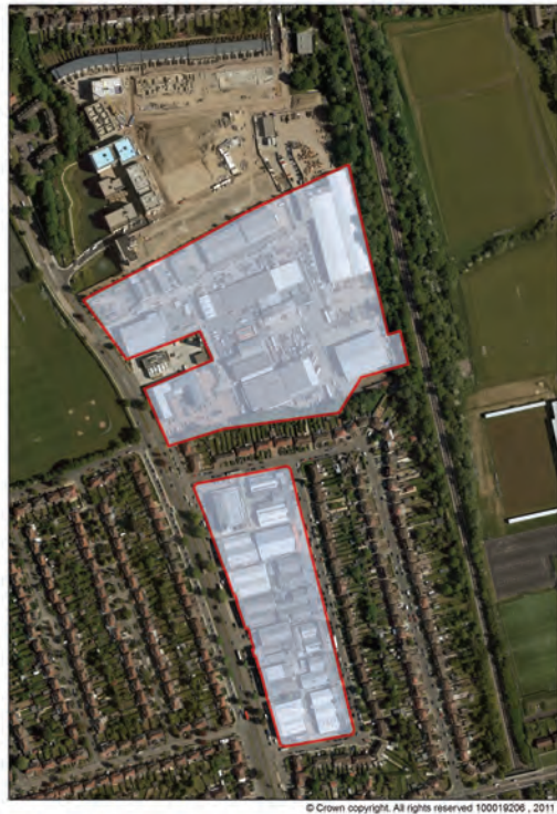
Picture 1.2 Proposed Extent of the Honeypot Lane Strategic Industrial Location - area to north removed
